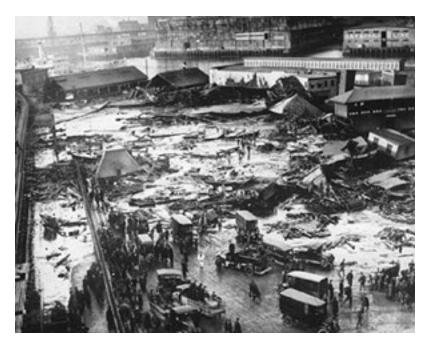
At 529 Commercial Street, a huge molasses tank 50 ft (15 m) tall, 90-ft (27 m) in diameter and containing as much as 2,300,000 US gal (8,700,000 L) collapsed. Witnesses stated that as it collapsed there was a loud rumbling sound like a machine gun as the rivets shot out of the tank, and that the ground shook as if a train were passing by. The collapse unleashed an enormous wave of molasses between 8 and 15 ft (2.5 to 4.5 m) high, moving at 35 mph (56
